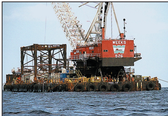
Crane getting ready to drop the bridge and ERS (Engine Recovery System).
